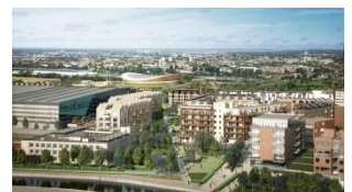
Public space through Phase 1 brings together the industrial Hackney Wick with the natural QEOP
