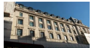
Regent Street retained Facade
