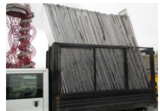
Polycarbonate cladding being taken away by Groundwork
